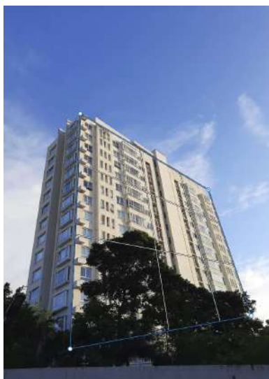
Picture 3: The quad created is now aligned with one face of the building.
